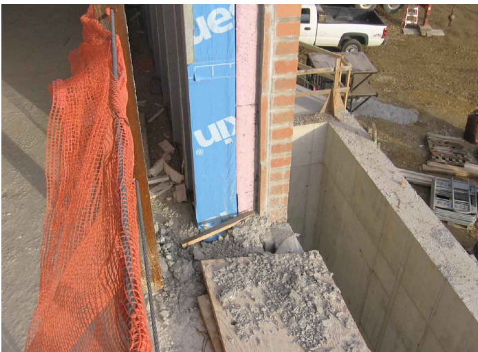
Example 1C: Jamb to sill intersection
