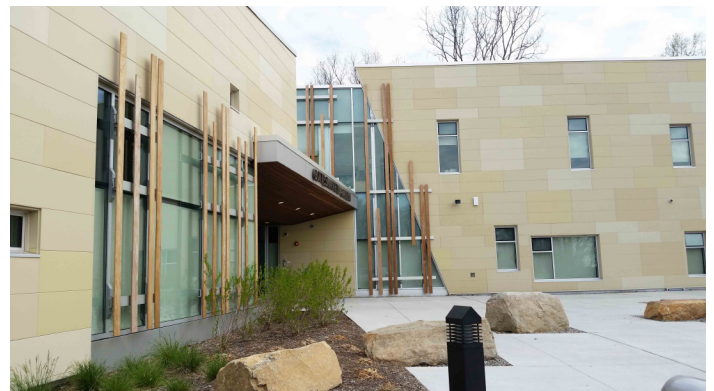
Figure I: Left and below: The glazing system can be engineered to accommodate different geometries as well as support the cladding material.
