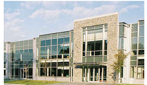
Figure C: Above and right: Specular painted finishes are applied to create depth and relief within the glazing assembly.
