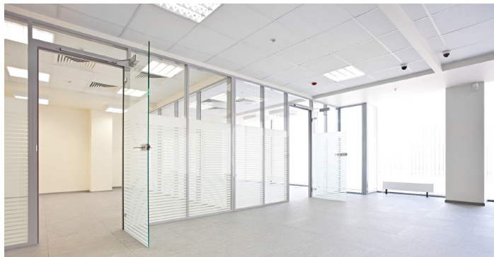
A framed system with mullions on all four sides of the lites
