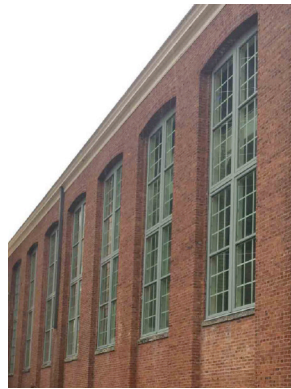
From left: J&J Museum before and after window replacement (images courtesy National Glass & Metal Co., Inc.); 1820 Rittenhouse Square replacement in progress: the black-framed double-hung windows were replaced with the gray-framed awning windows (image courtesy GMI Contractors, Inc.)
