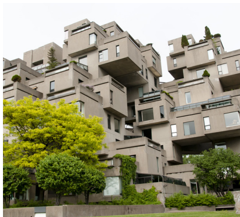
Energy modeling and design must consider all six sides of the enclosure (walls, roof, floors) as seen in Habitat 67 (image courtesy Fotolia)
