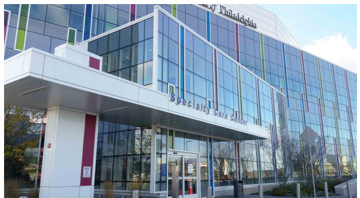
FIGURE 3: From top: Condition identified during construction as needing further review and assessment; testing to verify performance criteria; completed, high-performing glazing assembly
