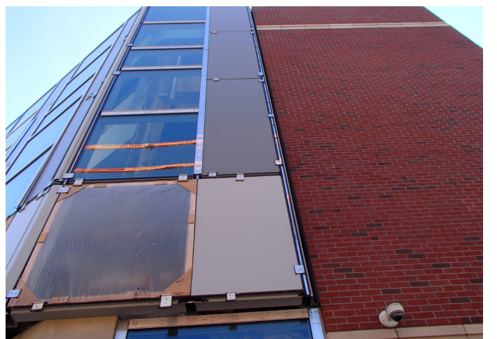
FIGURE 1: Left: Plan detail of a glazing assembly transition to masonry cladding; From top: Shop drawing detail of glazing transition to masonry cladding; proposed method for constructing an effective glazing assembly transition to masonry cladding; glazing assembly transition to masonry cladding as built; Top right: Completed glazing assembly
