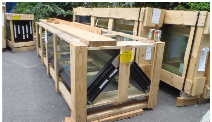
From top: Stock aluminum glazing stops for stick-built construction; shear blocks provide robust connection between vertical and horizontal framing; screw spline provides a direct connection between vertical and horizontal elements; unitized panels factory-crated and ready for installation
