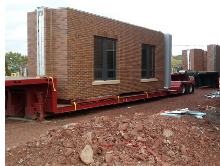
Above and left: Panelized wall detail: unit A (red) is inserted into the sill section (blue); pre-fabricated glazing assembly incorporated into a panelized exterior wall assembly; exterior wall panel staged at the site for erection
