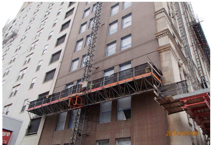
Image 8: Mast climbing work platform
