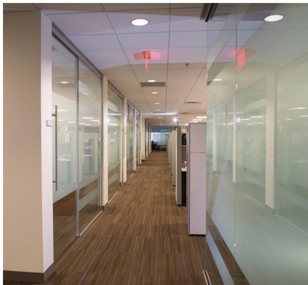
Right: demountable glass partitions at Lincoln Financial (Radnor, Pa.) by AGI member Reilly Glazing, Inc.
