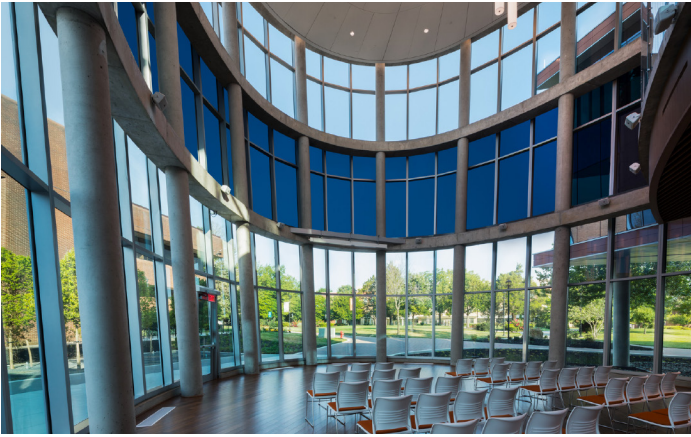
Dynamic SageGlass with the ability to change tint automatically.
