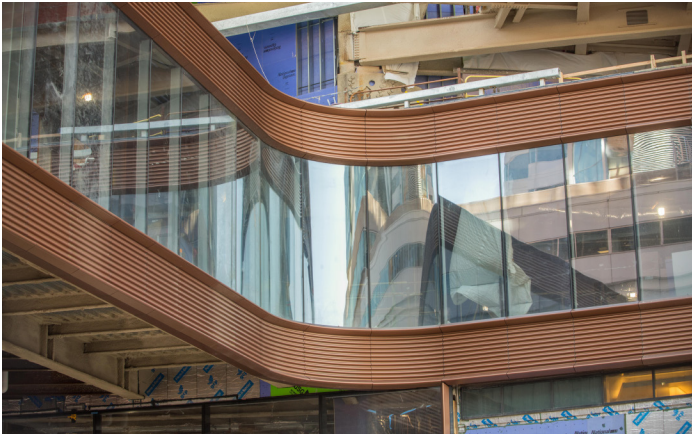
Detail of bent glass at Penn Medicine Pavilion (photo © Joe Garvin)
