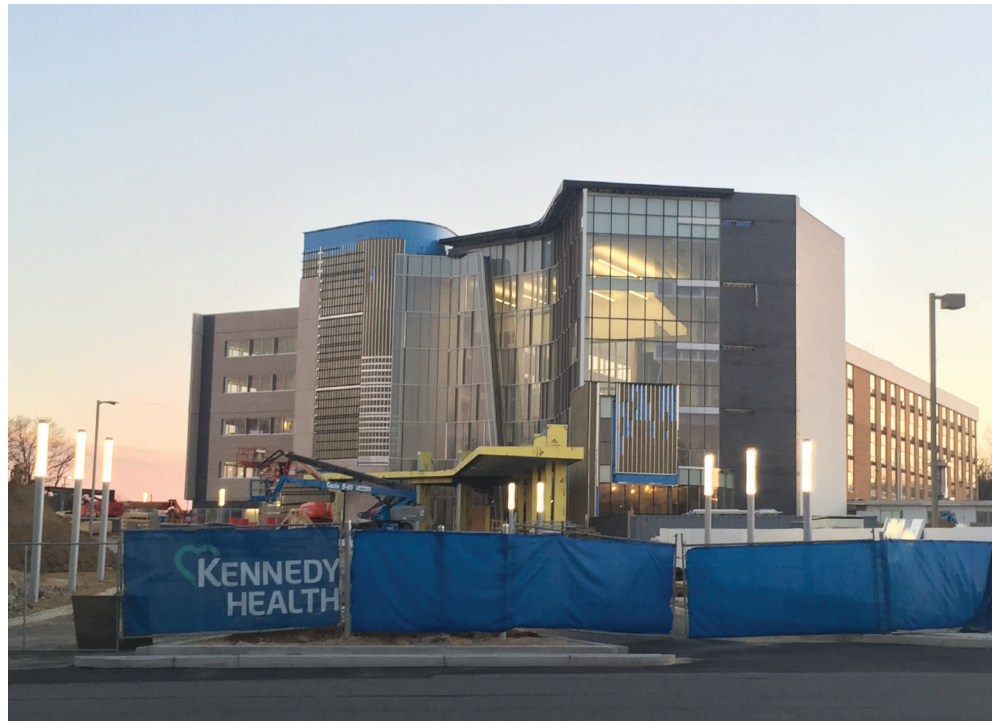
The curtain wall was completed in March; photo © Amanda Weko
