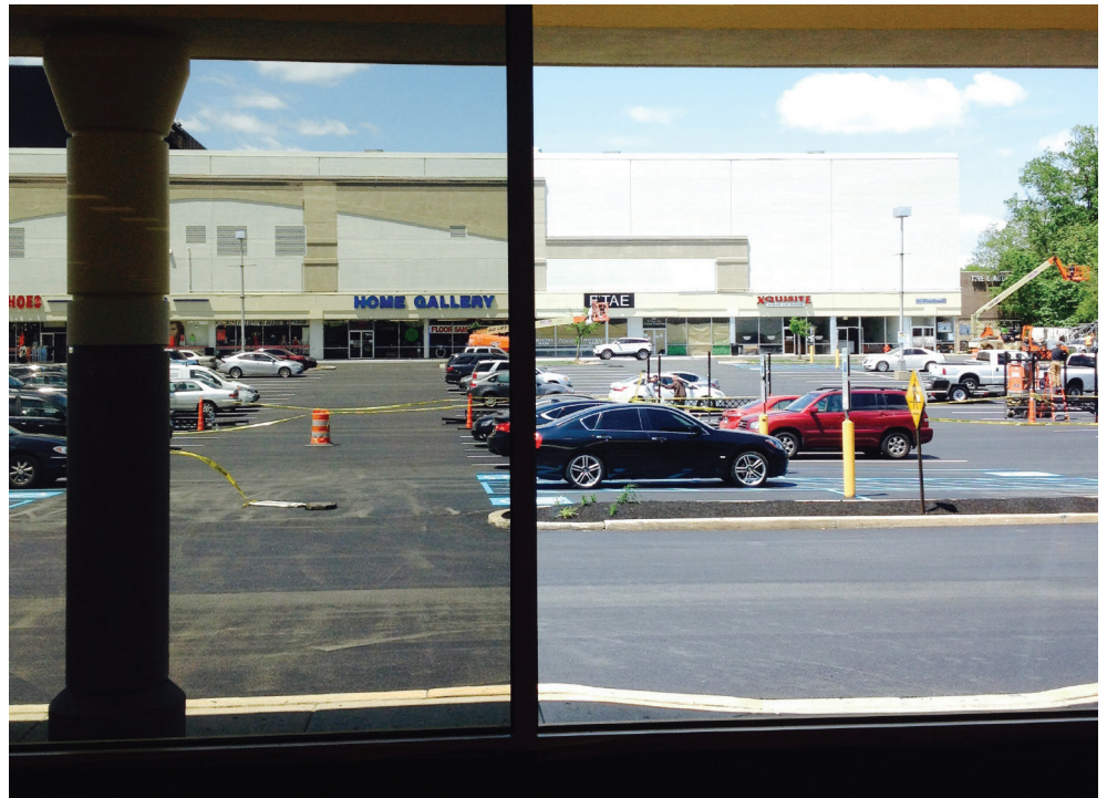
Storefront glass with (left) and without (right) solar control film (all images courtesy Eastern Solar Glass)
