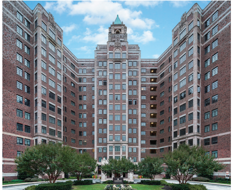
Alden Park Cambridge Building after renovation (photograph © Marc Harary, courtesy BartonPartners)
