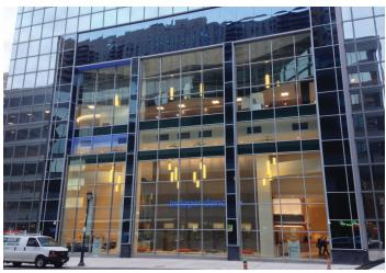
stainless steel cladding was fabricated to marry the existing steel to the new doors. Rabinowitz provided layout drawings for field constraints (an element not usually included in the scope) to help the general contractor make progress without waiting.
