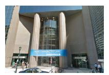
The structure within the large stainless-clad columns had to remain; new revolving doors were carefully fit into the space between the existing vertical steel.
