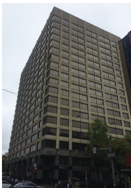
3535 Market Street before window replacement or exterior painting.
