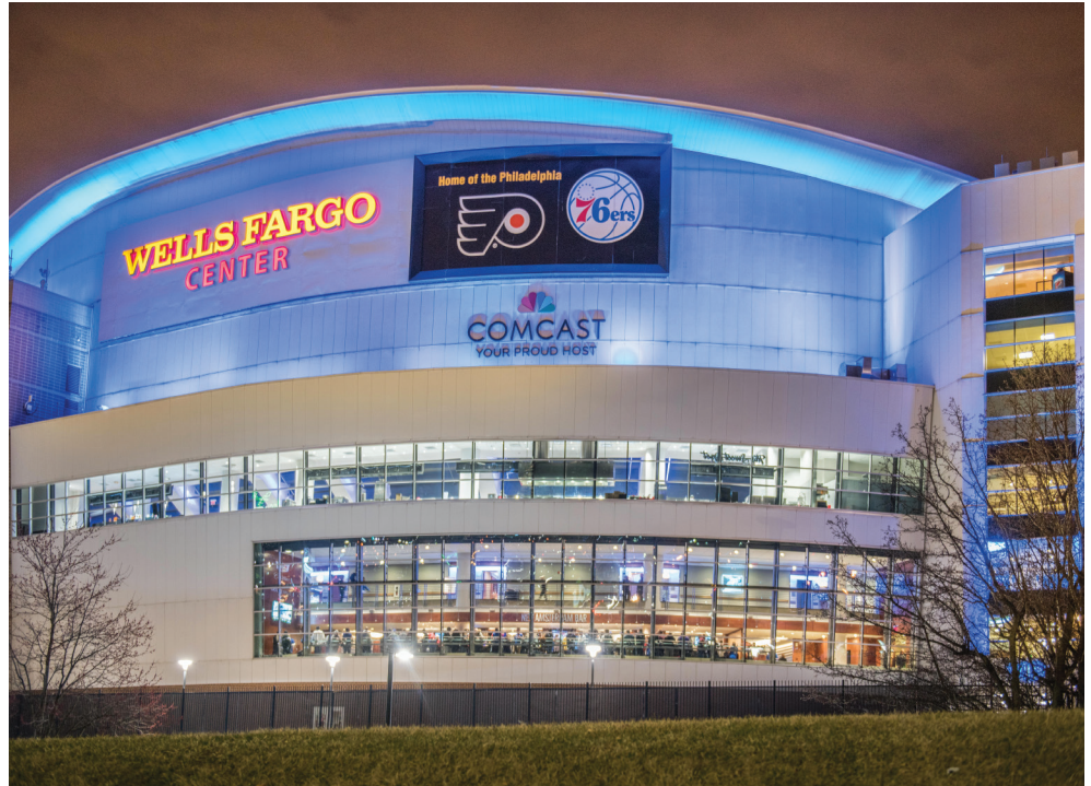
Rabinowitz Glass added the new upper band of curtain wall; photos © Joe Garvin except where noted
