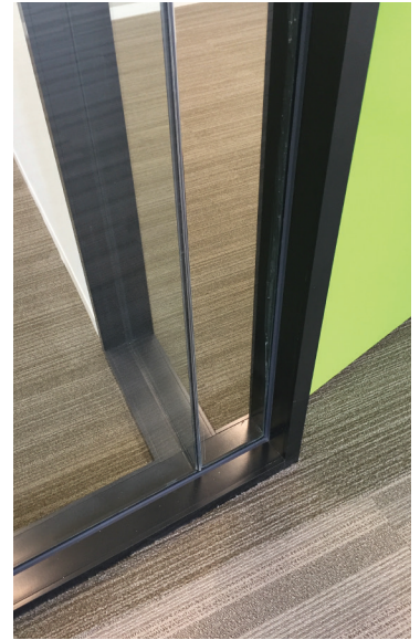
Left to right: conference room with back-painted glass (photo © Jeffrey Totaro), detail of butt-joined glass corner; detail of caulk and aluminum framing showing butt-joined glass detail and acute angle (final walkthrough photos © Amanda Weko)
