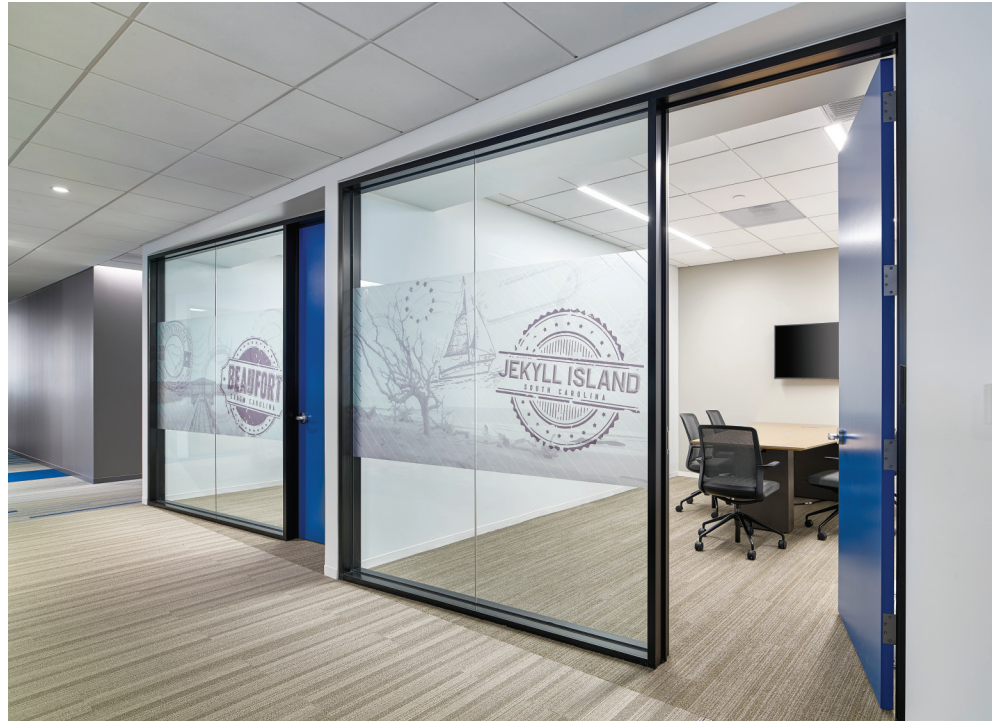
Meeting rooms with angled glass and aluminum partitions (photo © Jeffrey Totaro)
