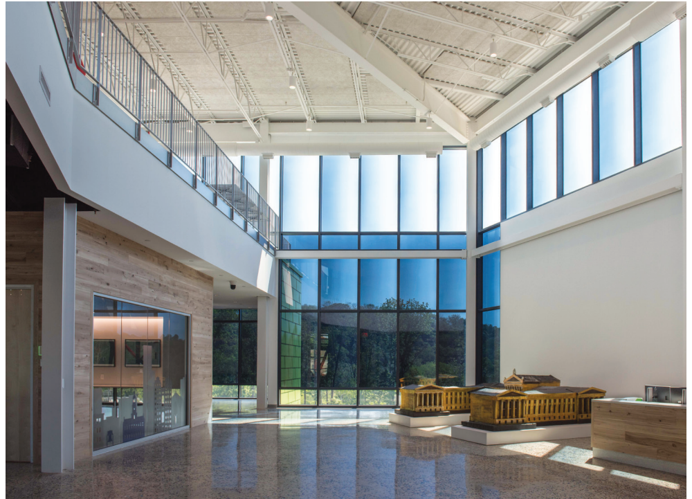
Lobby with central panes of electrochromic SageGlass set to shade (all photos © Joe Garvin)
