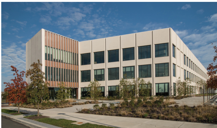
Clockwise from top left: exterior showing curtainwall with fins and punched openings; detail of main entrance with close-up view of wood-painted metal, Ipe fins, and both vision and spandrel glass; side view showing ripple effect of metal cap projections; corner view showing ribbon windows
