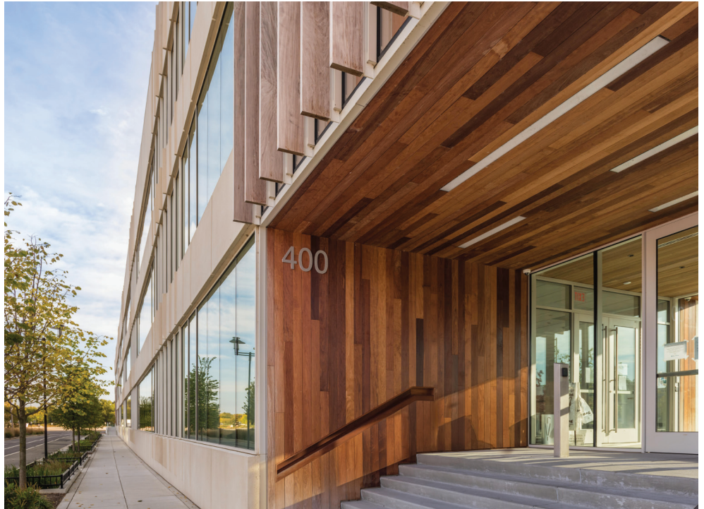
Main entry view showing detail of lpe fins and ribbon window projecting caps (all photos © Joe Garvin)
