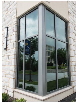
Both vision and spandrel glass was installed; the green-tinted spandrel glazing permits a regular fenestration pattern while masking production equipment and interior walls. Special posts were fabricated for where glazing connects at the building corner and entry.
