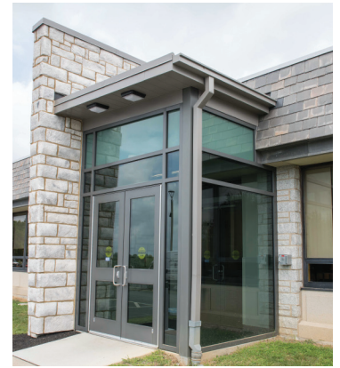
Both vision and spandrel glass was installed; the green-tinted spandrel glazing permits a regular fenestration pattern while masking production equipment and interior walls. Special posts were fabricated for where glazing connects at the building corner and entry.
