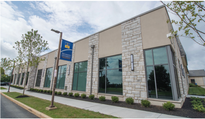
Both vision and spandrel glass was installed; the green-tinted spandrel glazing permits a regular fenestration pattern while masking production equipment and interior walls. Special posts were fabricated for where glazing connects at the building corner and entry.
