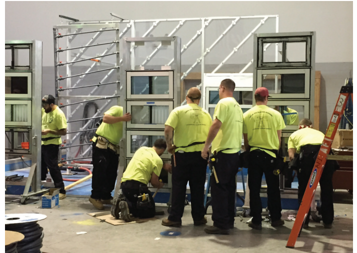
Top to bottom: Glazier Academy Cadets prepare curtain wall mock-ups for water testing; Philadelphia School Partnership grant being received by FTI (Philadelphia Mayor Jim Kenney at far left); cadets erect stick-built curtain wall section
