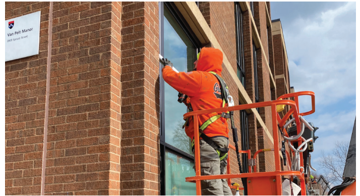
image © D&D Family Construction, LLC
