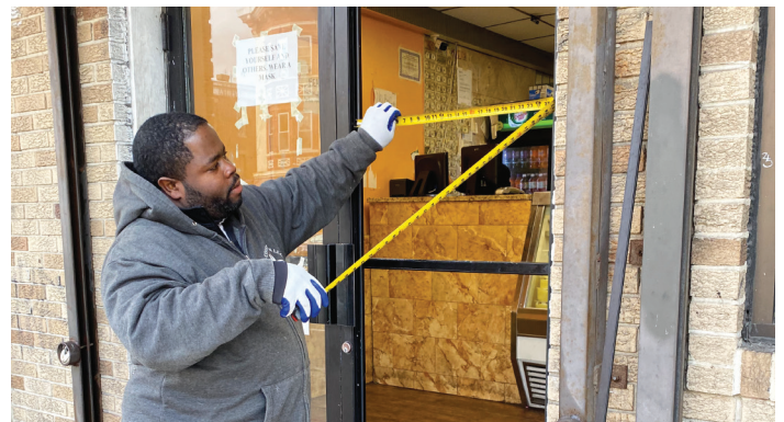
image © D&D Family Construction, LLC
