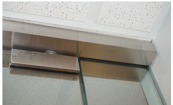
Below bottom: non-demountable, fixed interior glazing detail
